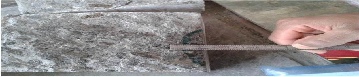
Fig. 16. Measurement of water penetration in concrete sample.
